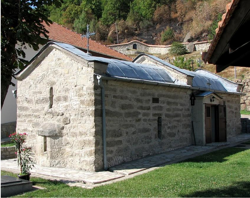
Fig. 1. The church building built in two stages of construction
